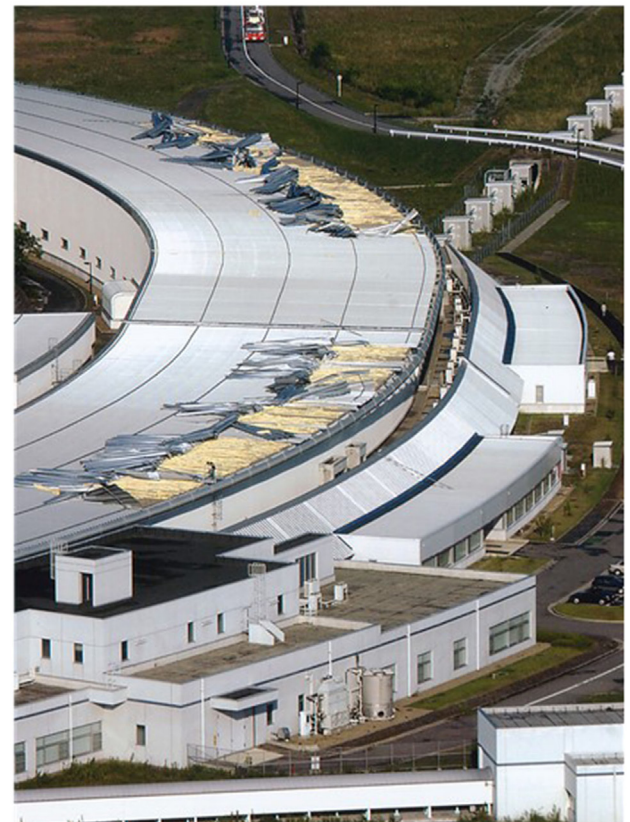
FIGURE 4 | Damage to two-layer folded steel plate roofing system of SPring-8, Riken, Hyogo, Japan, by Typhoon Chaba and Typhoon Songda, 2004 (by Kyodo: Tamura et al., 2005).
