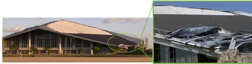
FIGURE 6 | Damage to steel roof sheets on a gymnasium in Kagawa, Japan, caused by Typhoons Dianmu, Namtheun, and Tokage, 2004 [courtesy of F. Nagao and H. Nishimura (Nishimura et al., 2005)].
