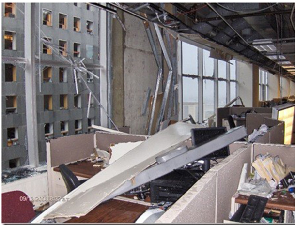
FIGURE 8 | Damage to a tall building in Houston, TX, USA, due to Hurricane Ike in 2008 (Brewick et al., 2009, courtesy of A. Kareem).
