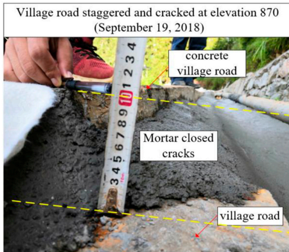
FIGURE 5 Deformation signs in the middle part entering the dry season.
