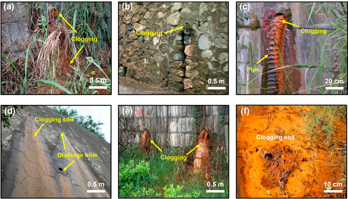
FIGURE 1 Inclined drainage holes with poor drainage and clogging problem: (A) red clogging soil with plants; (B) brown clogging soil; (C) soft drainage pipe with red clogging soil; (D) clogging materials after rainfall; (E) totally clogging drainage holes; (F) red clogging soil near the drainage holes
