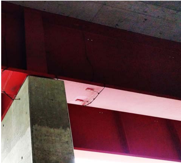
FIGURE 3 | Sensors B1 and B3 on the Venoge bridge (Credit: IMAC, EPFL).
