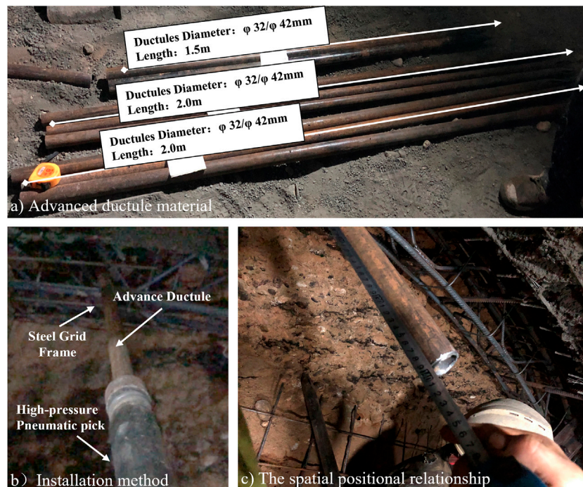
FIGURE 3 Schematic diagram of using small conduits and installation methods in the experiment.
