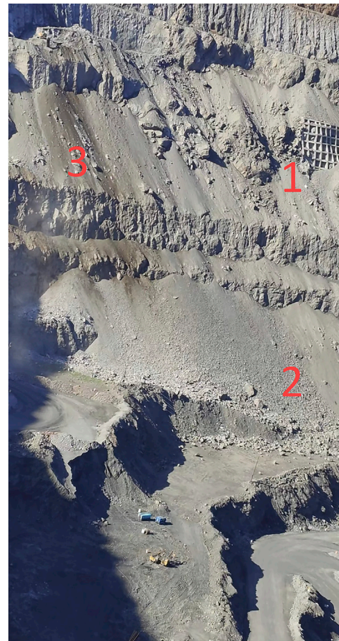
FIGURE 2 Extent of lateral slope collapse and the affected area.
