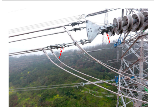
FIGURE 1 Transmission line bolt defects.
