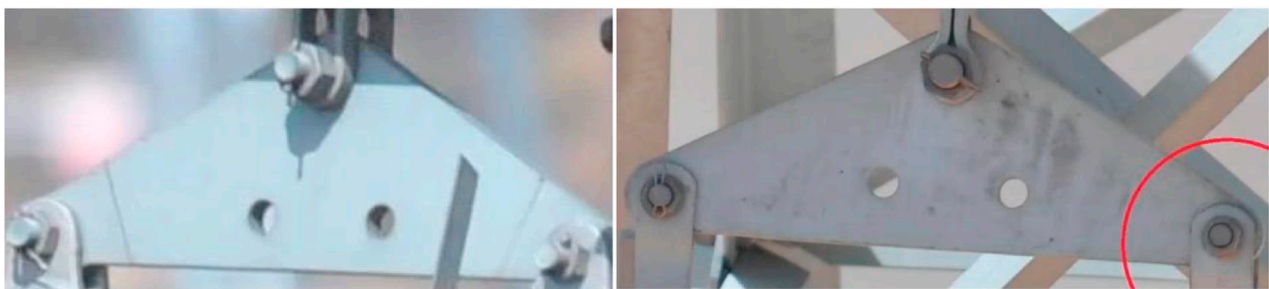
FIGURE 2 Transmission line bolts and their defects.
