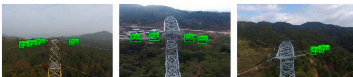
FIGURE 6 Example of fitting defects.
