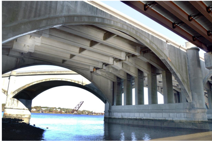
FIGURE 1 | Overview of a typical PSC girder span of I-195 WB bridge over Seekonk river.
