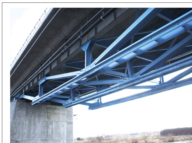
FIGURE 4 | Bottom view of the extreme span—visible details of the added structure during the renovation; from Olaszek (2015) permission was granted by The Committee on Civil Engineering and Hydroengineering of the Polish Academy of Sciences.
