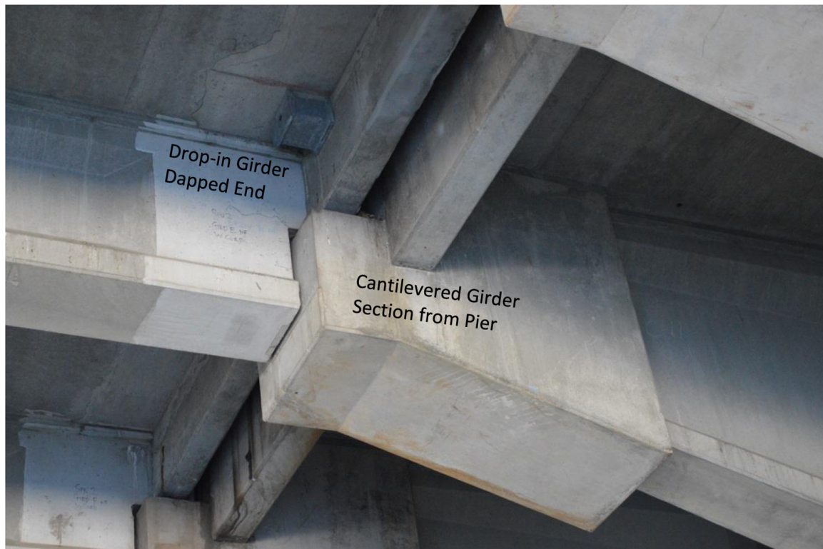
FIGURE 2 | Dapped end of drop-in girder supported by cantilevered girder section from pier.
