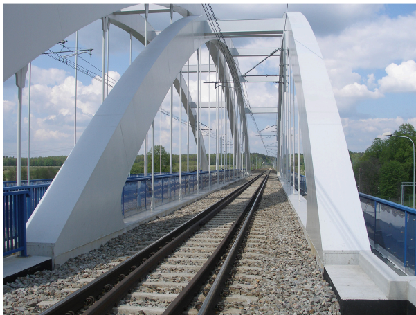
FIGURE 12 | View of the bridge from the railroad level—visible hangers made from steel bars.
